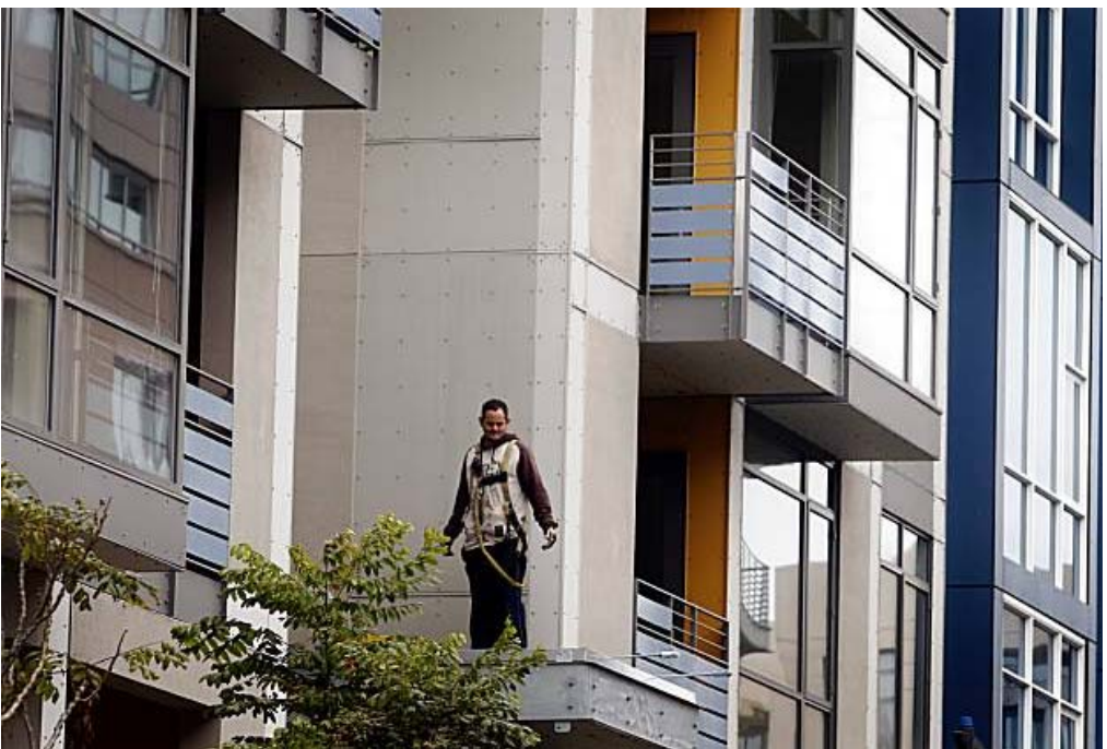
Construction workers add finishing touches to Mission Walk on Berry Street.
